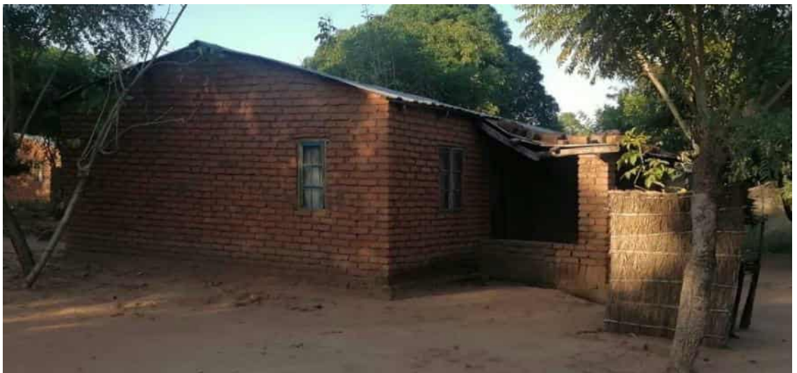
Figure 7: Burnt Brick, Earth Floor and Iron Roof House
