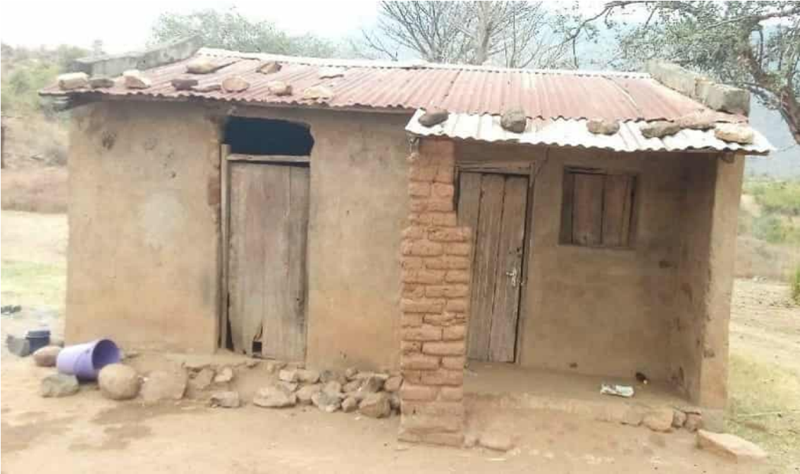
Figure 9: Burnt Bricks, Cement Floor, Plastered, Corrugated Iron Sheets House
