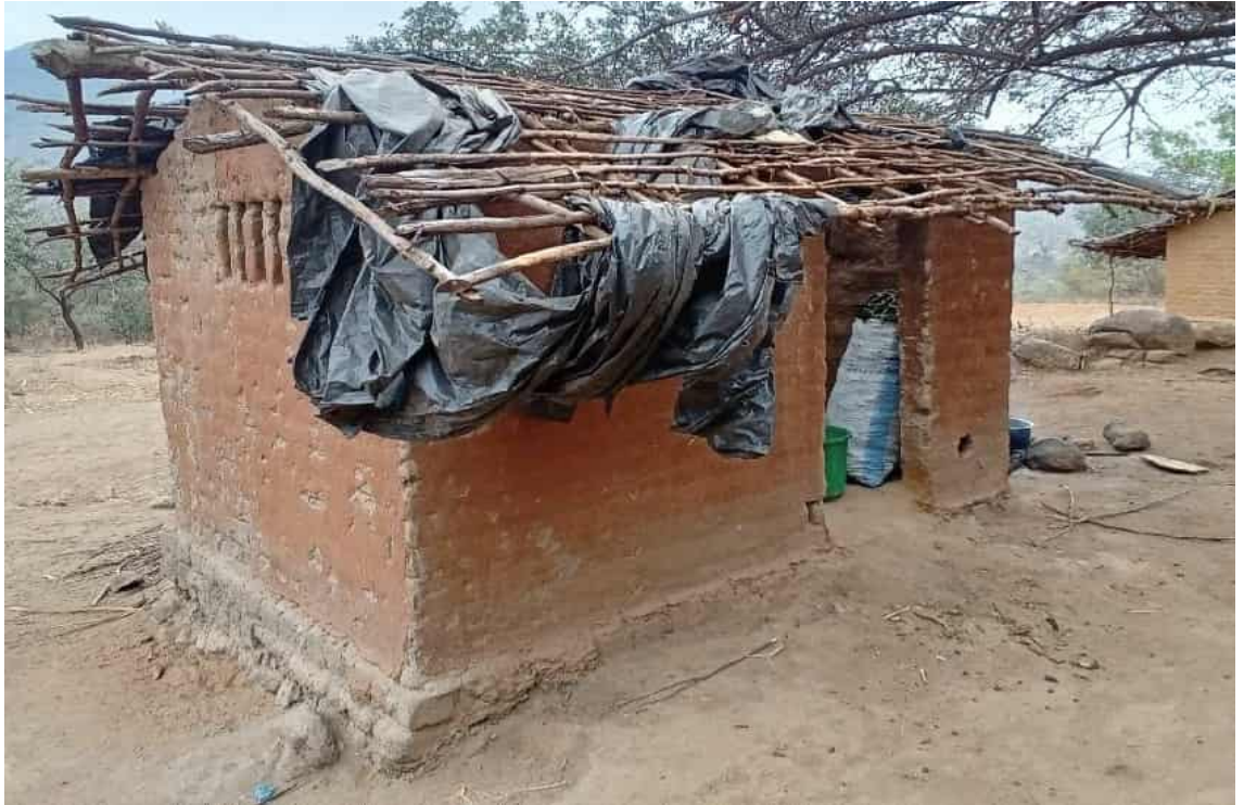
Figure 19: Burnt Brick, Earth Floor and Plastic Roof House
