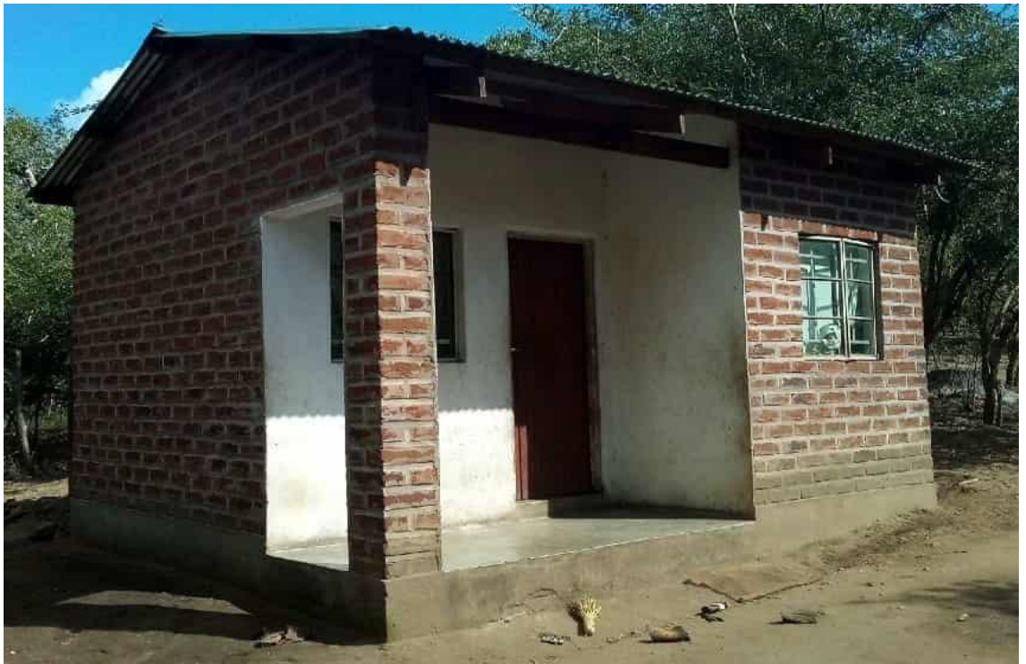
Figure 14: Burnt Brick, Cement Floor, Plastered and Iron Roof House
