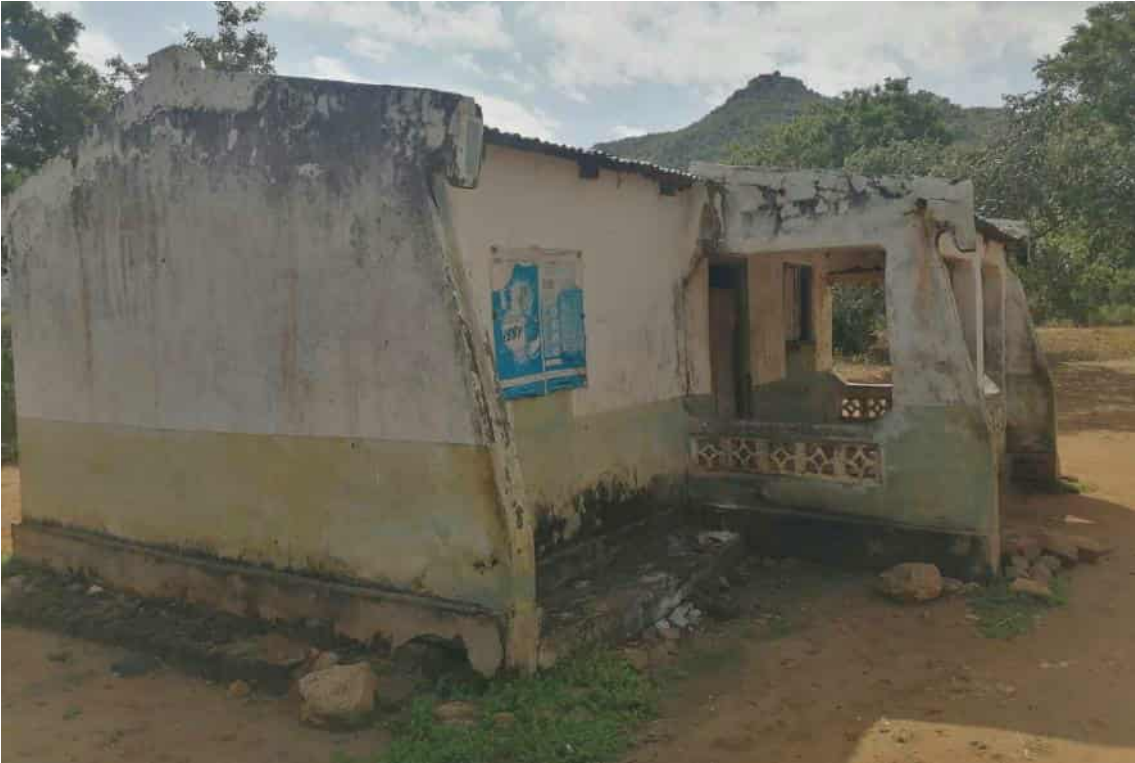
H8 Burnt bricks - cement floor - plastered inside and outside - corrugated iron sheets
