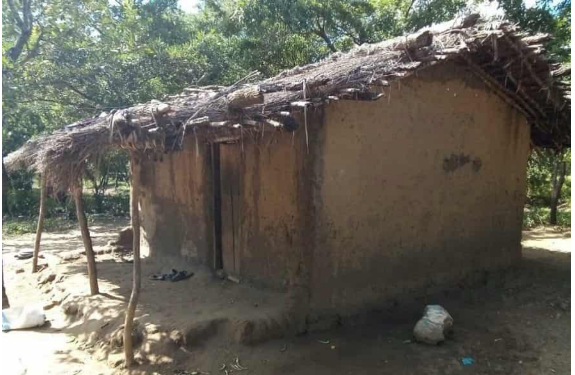
Figure 13: Sundried Brick with Mud Mortar, Earth Floor, Grass Thatched House
