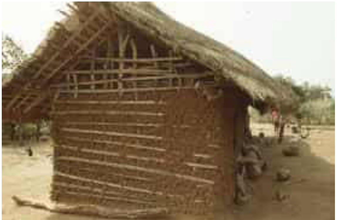
Figure 4: Mud and Wattle Structure
