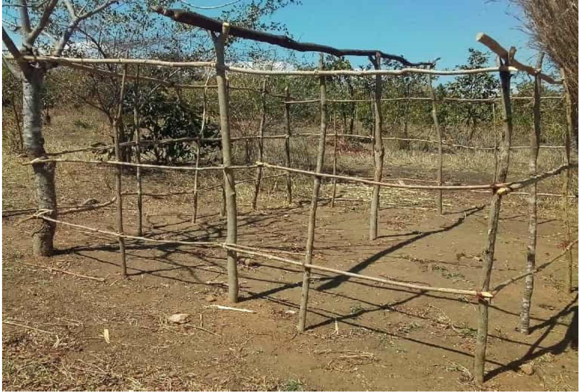
Figure 16: Wooden Poles House
