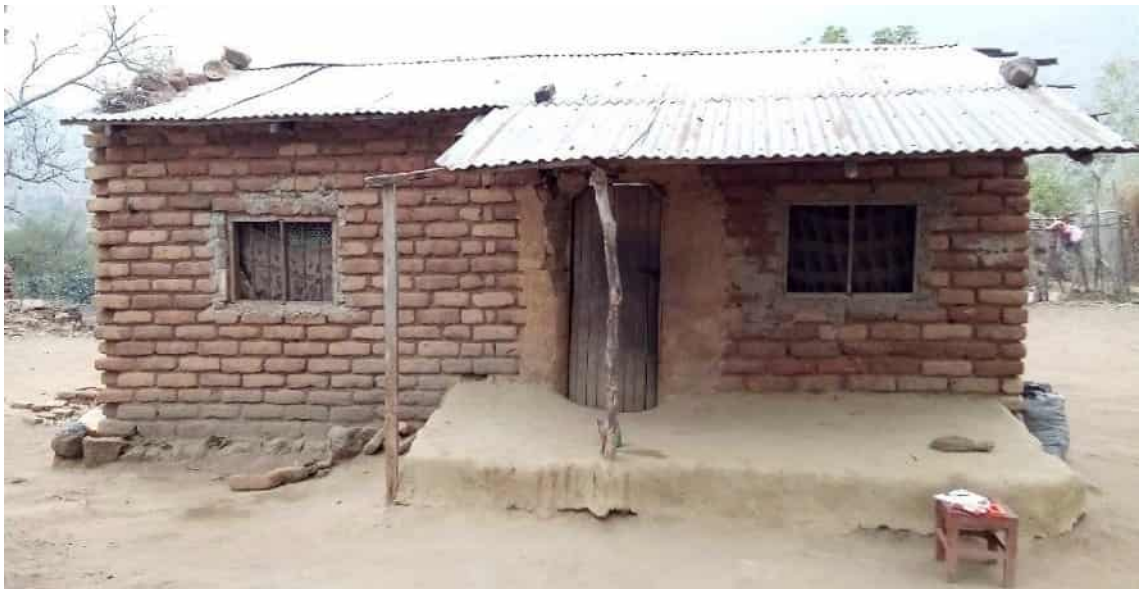
Figure 12: Stone Walls with Cement Mortar, Concrete Floor, Corrugated Iron Sheets House
