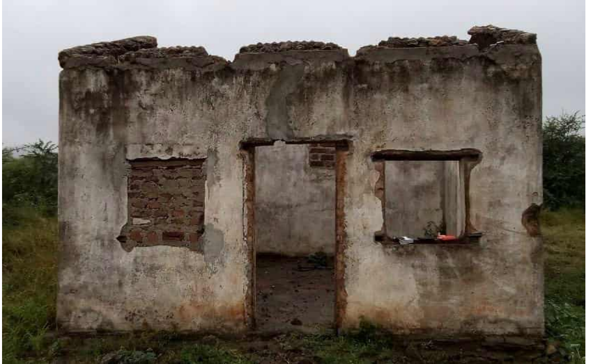
Figure 11: Burnt Bricks, Cement Floor, Plastered, Painted House
