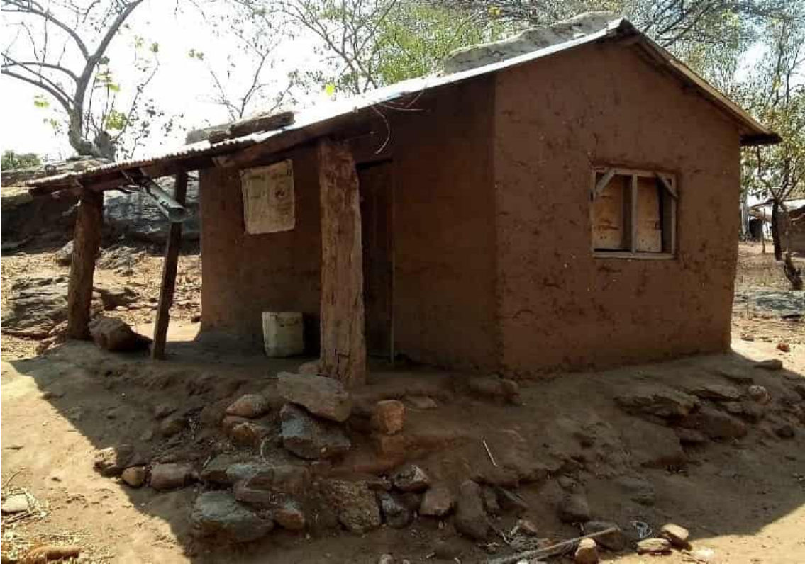
Figure 17: Sundried Brick with Mud Mortar, Mud Floor, Iron Roof House
